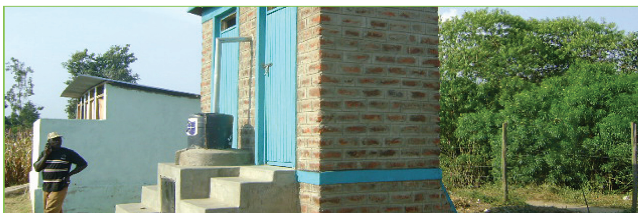
Complete Urine diverting dehydrating toilets (UDDT) in Kyaemba Primary School, Mumias.
