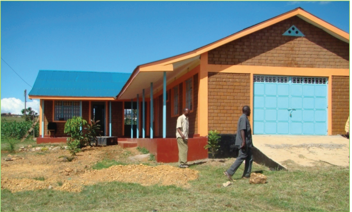
An appropriate building technology center constructed using Stabilized Soil Blocks (SSB) in Kakamega.
